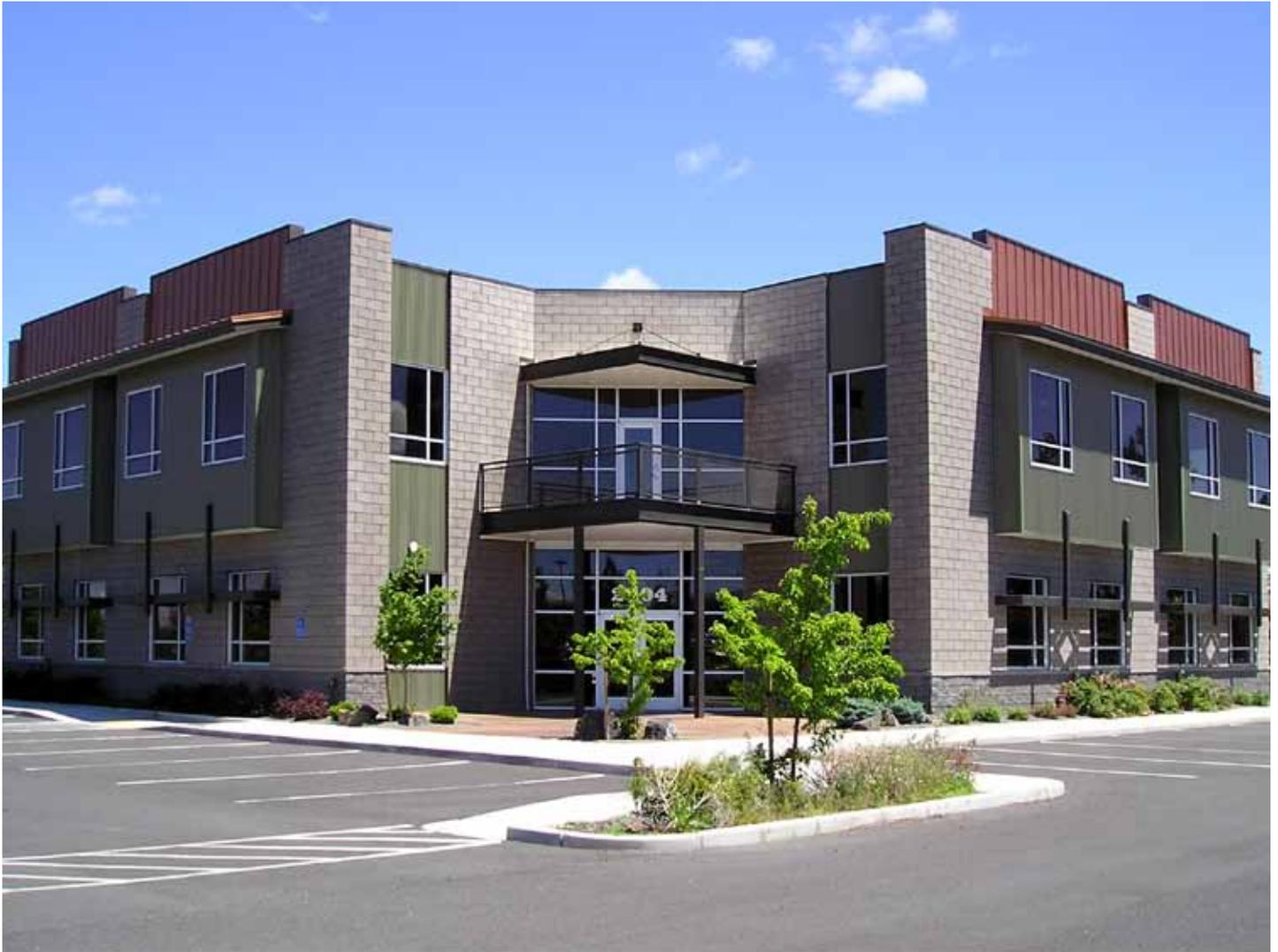
This 13,000 square foot Class A office building was designed and built for Diamond Built Homes, a multi- and single-family residential builder/developer based in Redmond, Oregon. Exterior materials combine steel and concrete with Insulated Concrete Form construction.
